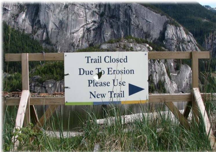
Coastal erosion at Squamish Oceanfront Peninsula, 2014
